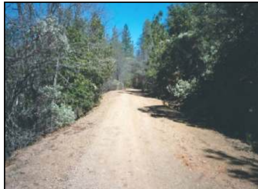
Waterman Road Showing Brush Encroachment
