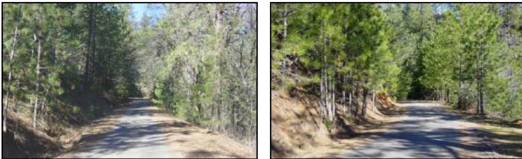
Skyline Drive showing over grown conditions
