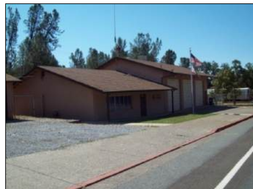
SLFPD Fire Station
