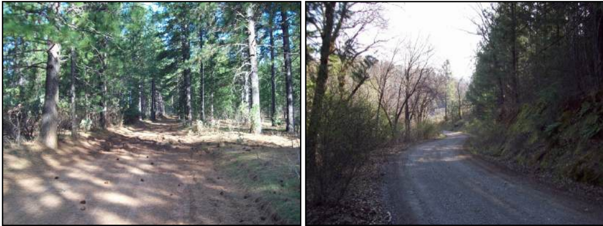
McCandless Gulch Road Fuelbreak: Note dense brush and trees up to the edge of the road.
