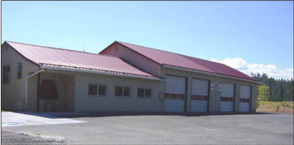
Old Station volunteer firehouse
