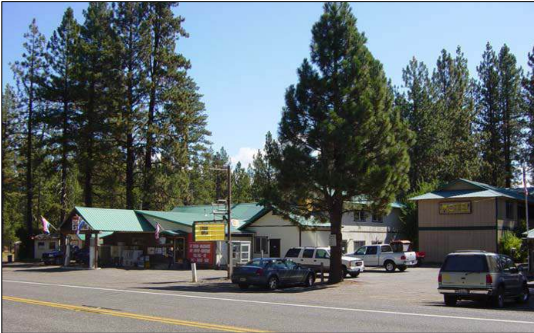
Hat Creek Store, Old Station
