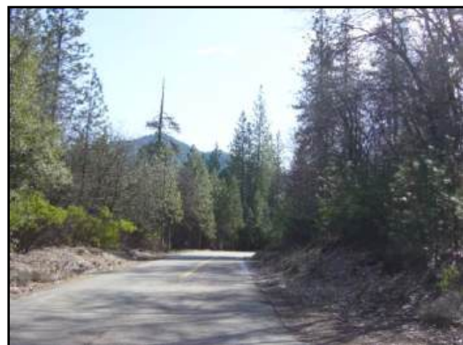
Mears Ridge Road north of the intersection with Sims Road.
