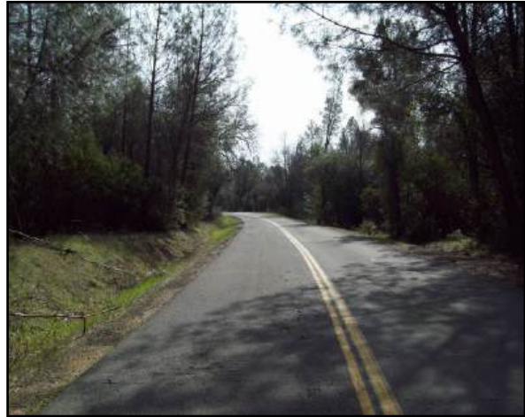
Rainbow Lake Road – note heavy tree and brush growth to edge of road.
