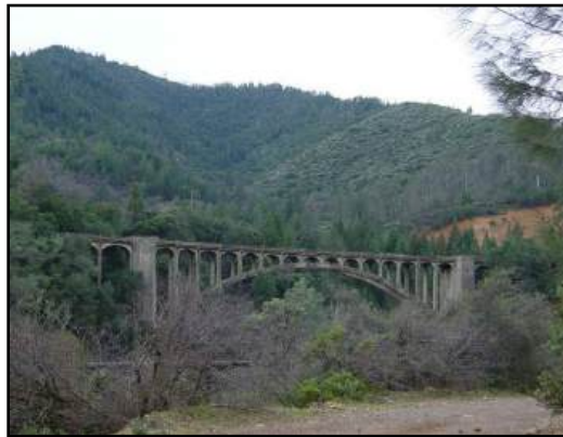
Dog Creek Bridge
