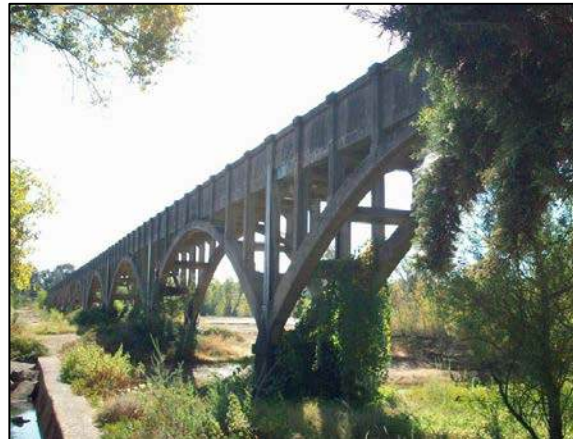
Anderson-Cottonwood Irrigation District (ACID) aqueduct is a Historical Place of Interest
