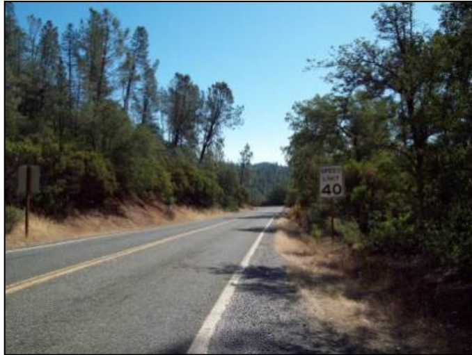
HWY-151. Note dense vegetation
