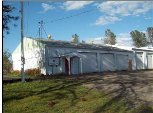
Oak Run Volunteer Fire Department Station
